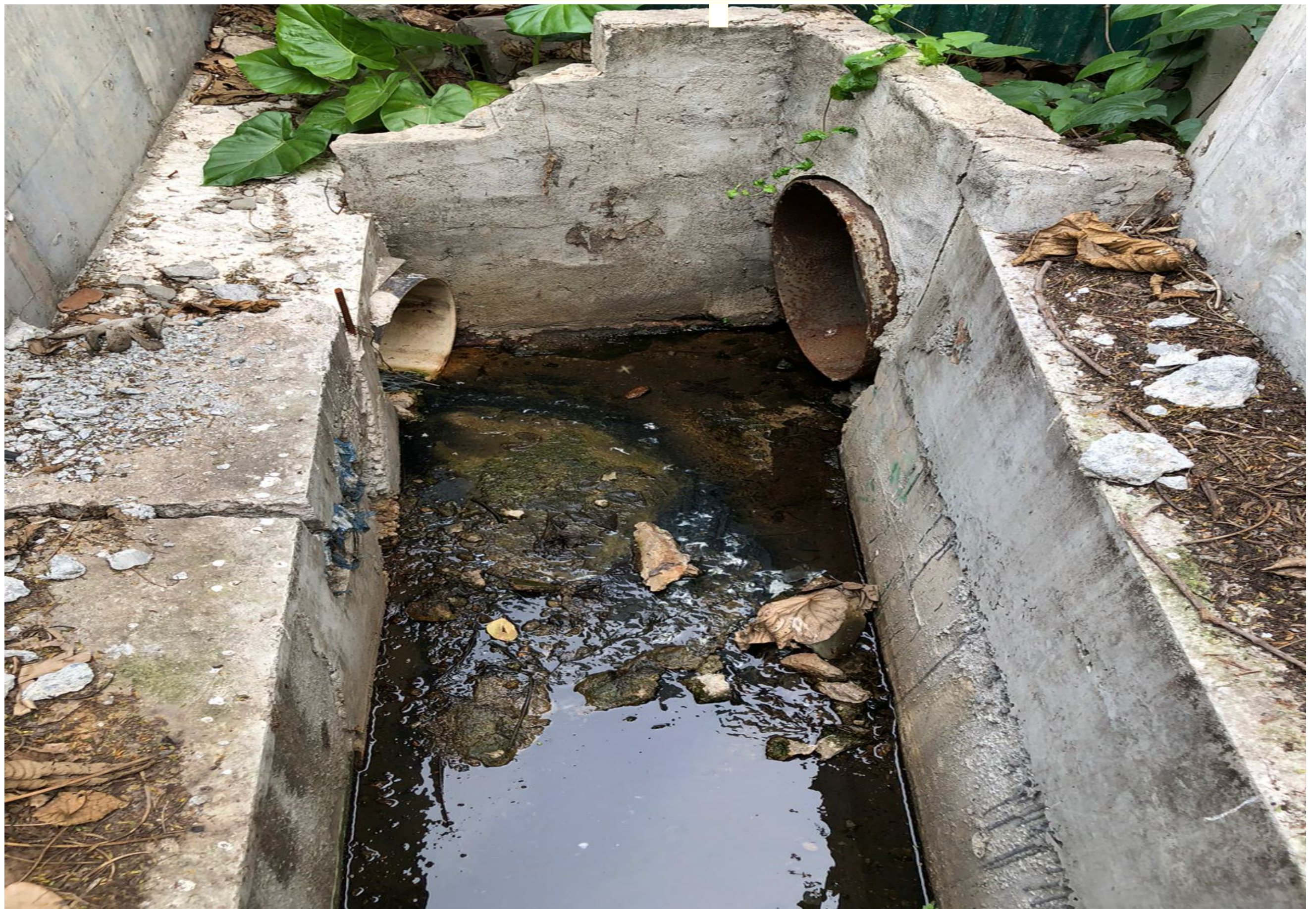
VIEW 2: FINAL DISCHARGE FROM EXISTING 400UPVC
